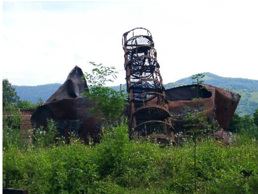
Picture 3: Destroyed heavy oil tank, right next to the Theiss
