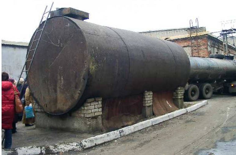
Picture 14: Storage facility
