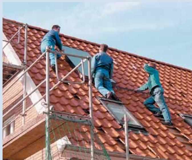
Montage Solaranlage in Oldenburg
