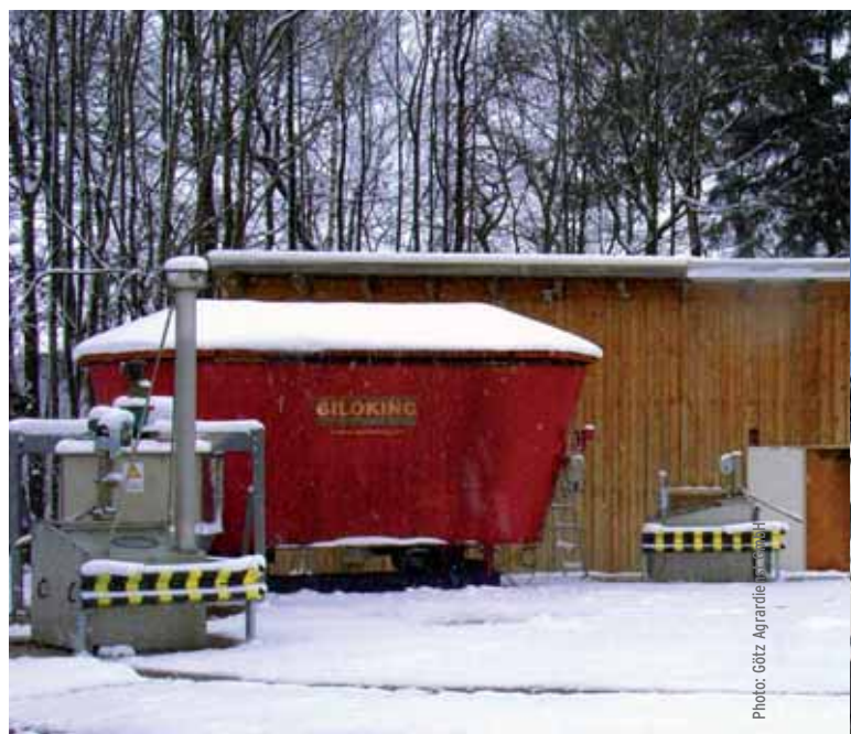
Biogas installation for renewable raw materials...
