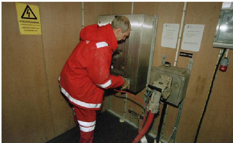
Picture 35: Supply of electricity for ships by means of a cable connection in port
