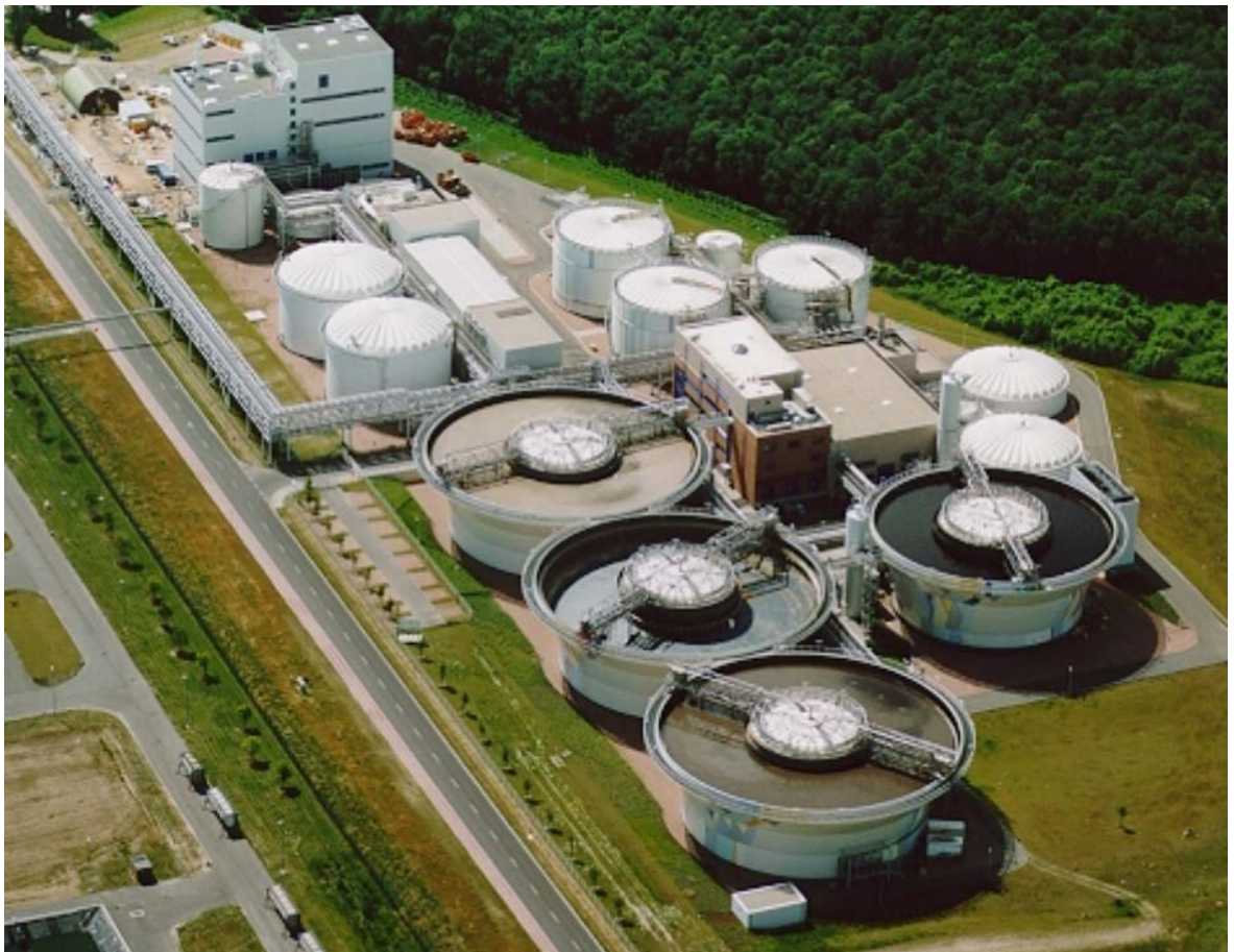
Figure 14: Joint WWTP Bitterfeld (above-ground bioreactor – population equivalent =453,000) (pilot project of the BMU for the joint handling of domestic wastewater and industrial chemistry wastewater)[5]
