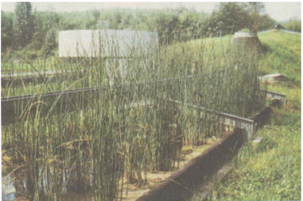
Figure 23: Root system treatment plant [22]
