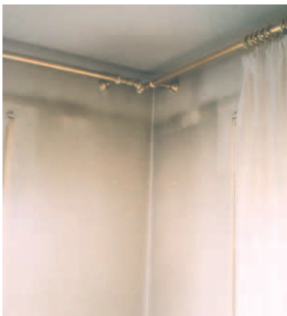
Black soot deposition occurred in this room six months after decoration work.
