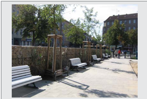
Photo 1: The gabion wall protecting the area with 3dB(A) against the road traffic noise (Carla Schlösser).
