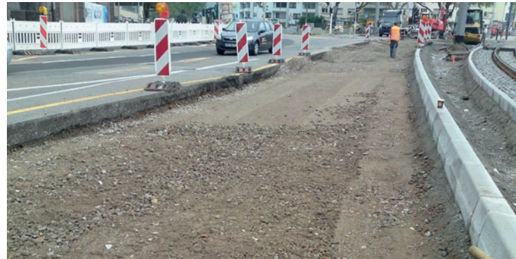
Installed and qualified quality-controlled frost protection layer from the material cycle
