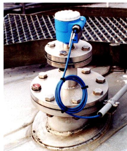
The filling level is the height of a liquid substance above a reference height. The maximum permissible filling level is the level which prevents the tank/container from being overfilled. There is still no design up today which fulfil all application- and safety-relevant requirements.
