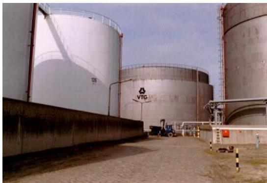
Flat bottom tanks in secondary containment: The vertical walls of the secondary containment are visible in the picture.
