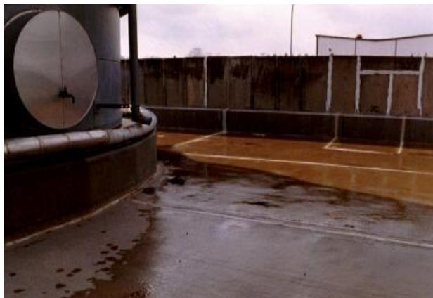
Flat bottom tank in a renovated secondary containment: The floor of the secondary containment and the lower part of the vertical wall surface is tight and resistant towards the storage environment. The upper part of the wall surface is also renovated and is for retaining fire-fighting water or foam. The flat bottom tanks are provided with a double bottom. The space between the double bottoms is being monitored for leaks.
