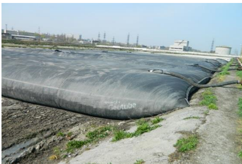
Storage of sludge in the central wastewater treatment plant of the capital Chisinau (Geotubes)
