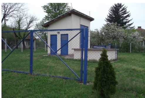
Small water supply in Tornjoš village
