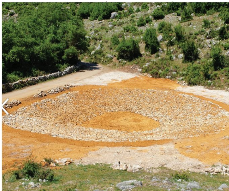
Figure 11: Construction of a dew pond in the village of Bzhetë, Shkrel, Malësi e Madhe, Albania (2021) (Source: GO2Albania, photo by Liridona Ura)
